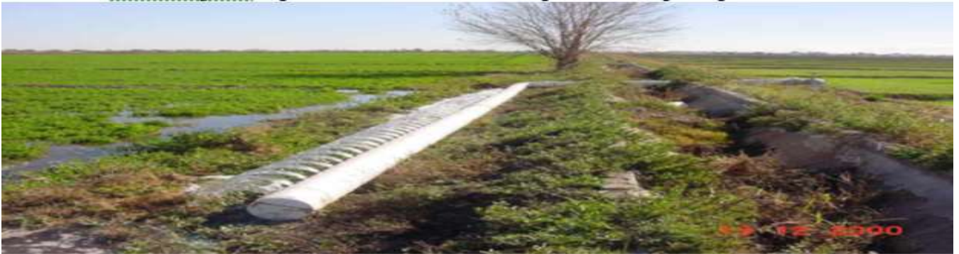
Figure.2. Plastic gated pipe for furrow irrigation
