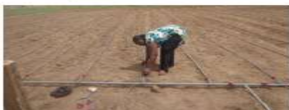
Plate 3: Connecting lateral pipes
